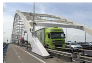
Merwede bridge closed for all heavy trucks!
